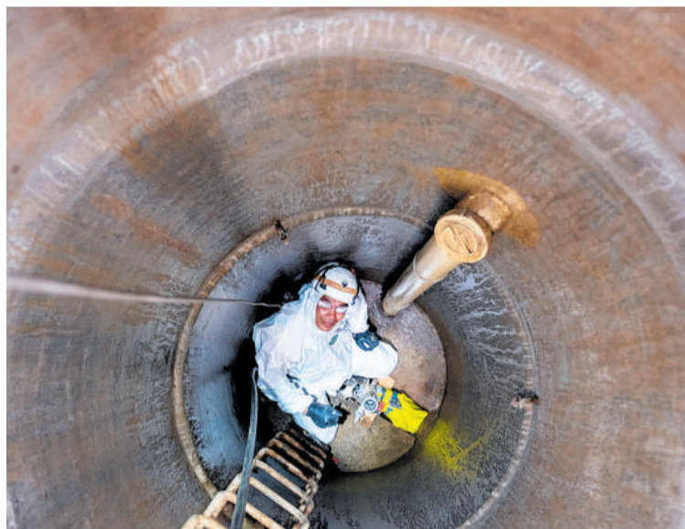
A crew member works on relining 6.2km of wastewater pipes in Beachlands and Maraetai.
