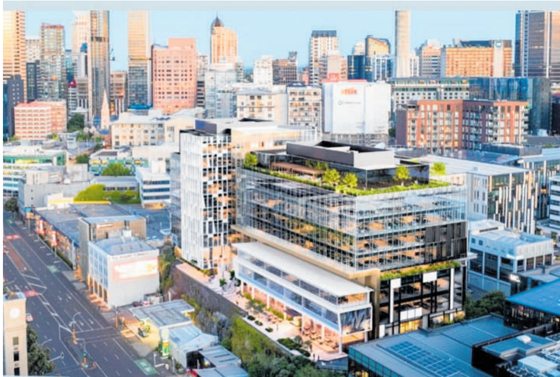
Mansons TCLM is building an 11-level twin-block project, connected via a central atrium on Graham St.
