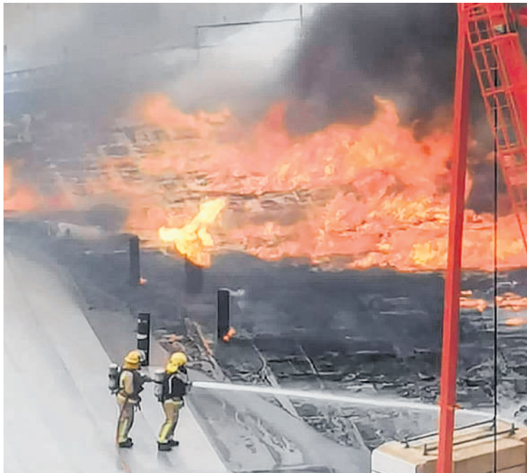
The 2019 fire at the International Convention Centre.
