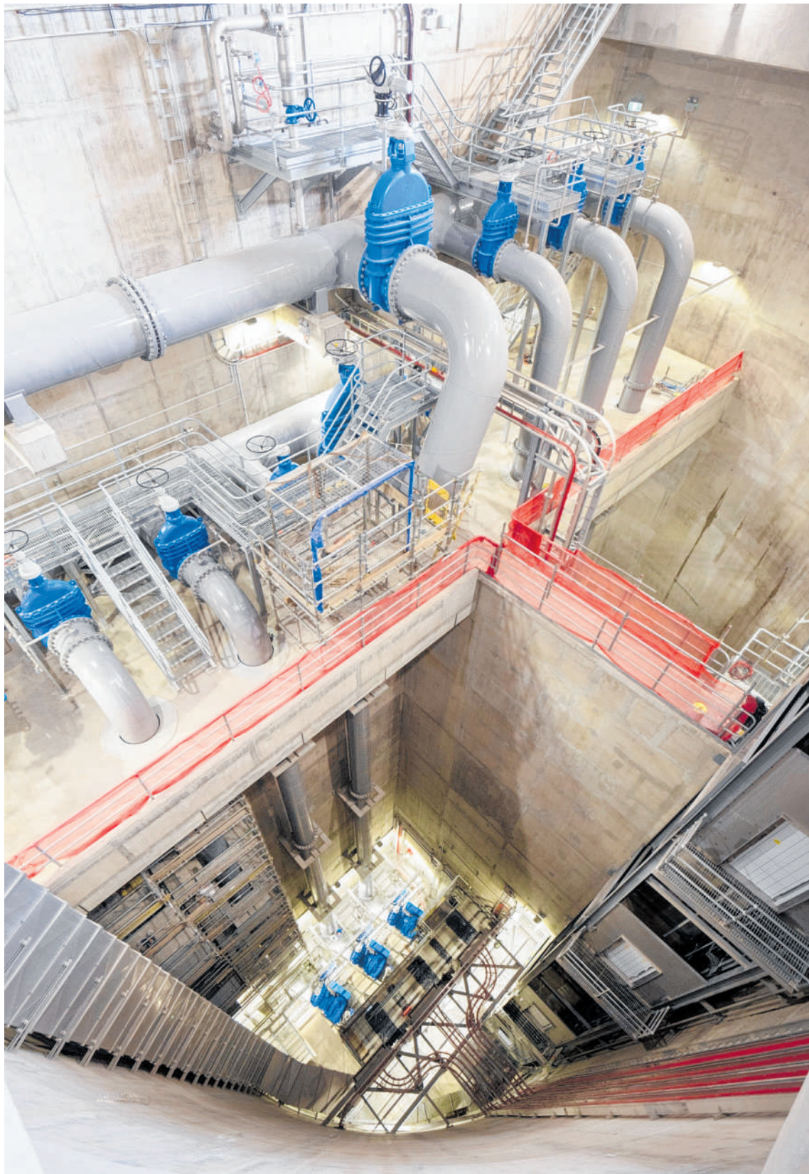
A new pump station at Watercare's Māngere Wastewater Treatment Plant takes flow from the Central Interceptor.
