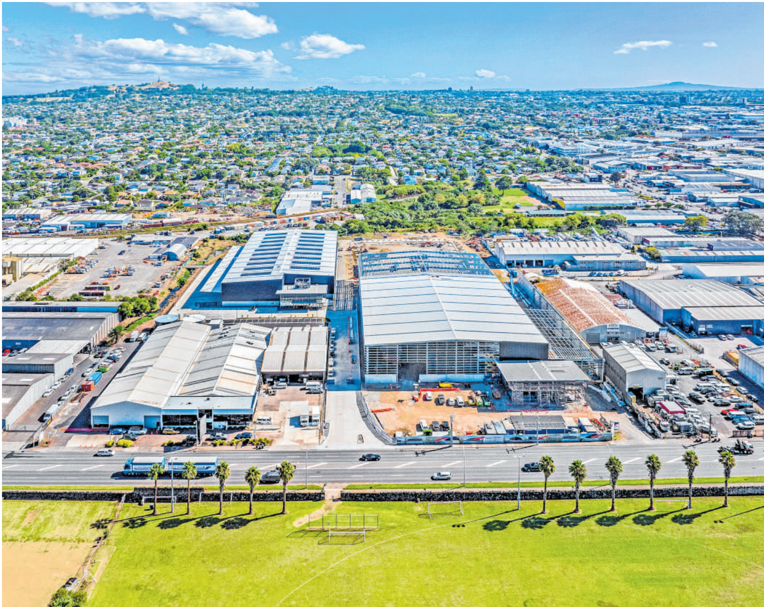
At 224 Neilson Street, Auckland, Argosy is developing a $100 million industrial park
